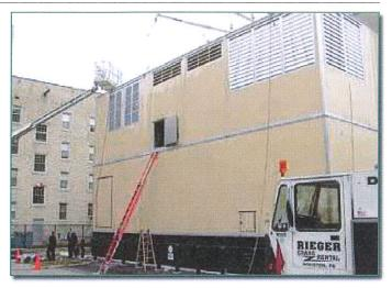
This 55 dB(A) reduction enclosure for a 1.8MW Diesel generator set is for a telecommunications facility. This is may be the quietest manufactured enclosure system for a 1.8MW diesel installation in the U.S.—achieving a third-party certified 45 dB(A) noise level at 50' in any direction. Pritchard Brown was the only packager contacted that was willing to tackle the project.
